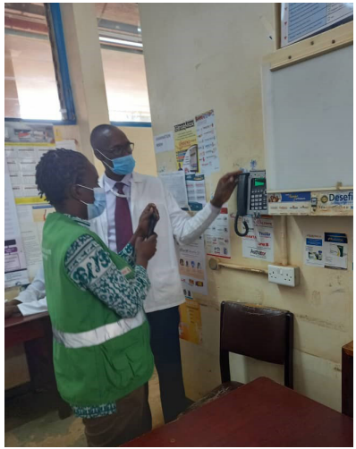
The national EMS coordinator testing the functionality of the installed deskphone at Mbale RRH.
